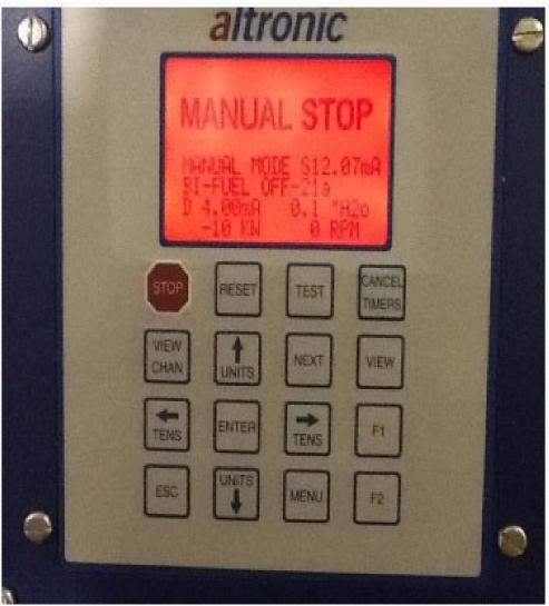
LEL Detection on each Gas Train is in place to shut off incoming gas to the Motor Shed and Boiler, If the LEL gauge is tripped it will show warning lights and the Altronic Panel will show Ch. 14 Gas Detection. Any gas leaks MUST BE Repaired before resetting Fuel Valve
