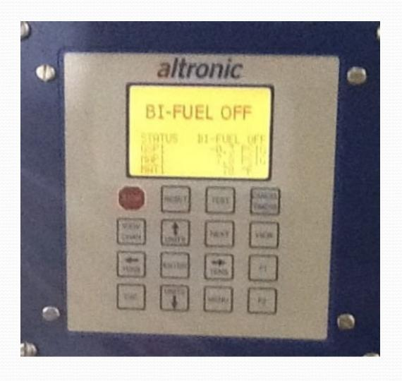
Power On Red Light On with Red Screen, Unit has Faulted Out and has Shut Down, Record Fault and Time, Push Reset If Fault Continues Turn Power Off, Close Ball Valve and Call ECO-AFS
