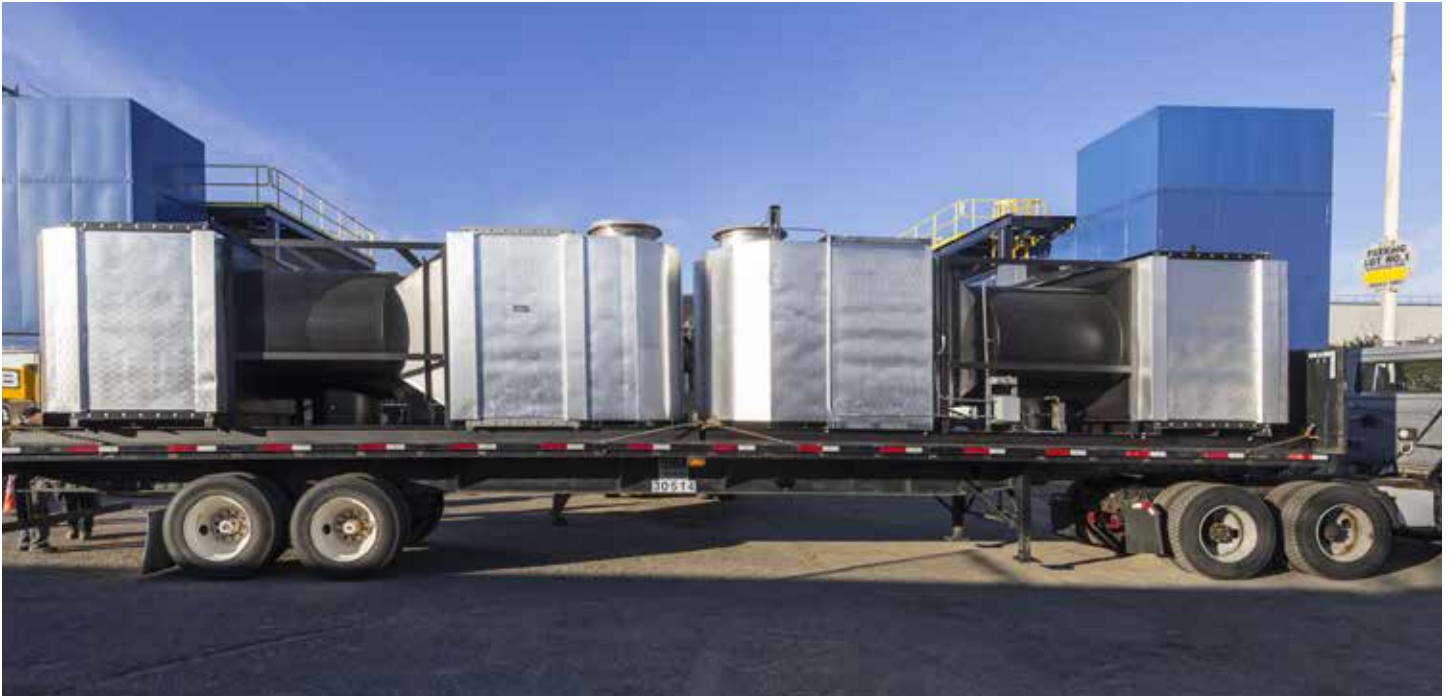
Two factory assembled CompactSCRT systems arriving at the jobsite. A single crane lift per unit eases installation.
